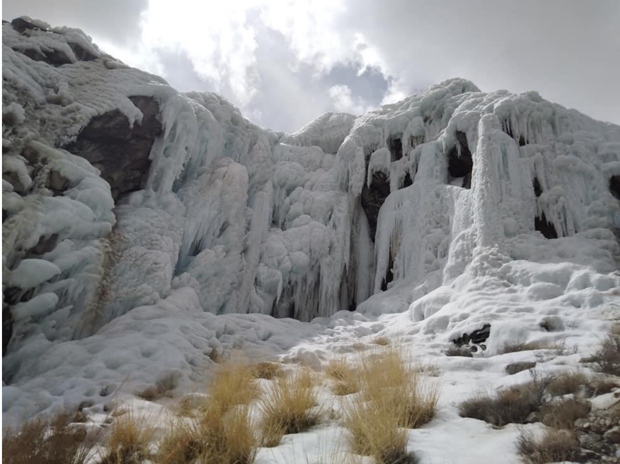
Figure 3: The Artificial Glacier constructed by the villagers
